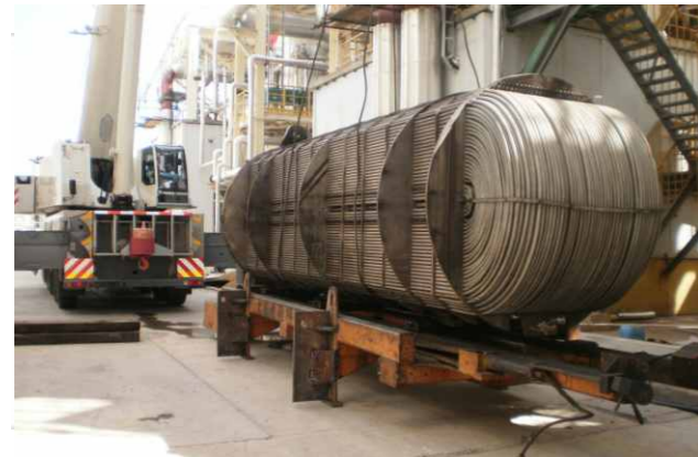
U型管换热器 U-tube heat exchanger
